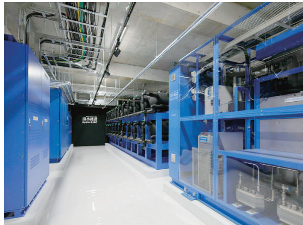
Hydro Q-BiC® Hydrogen Energy Utilization System for Buildings * Hydro Q-BiC® is a registered trademark of Shimizu Corporation in Japan.
