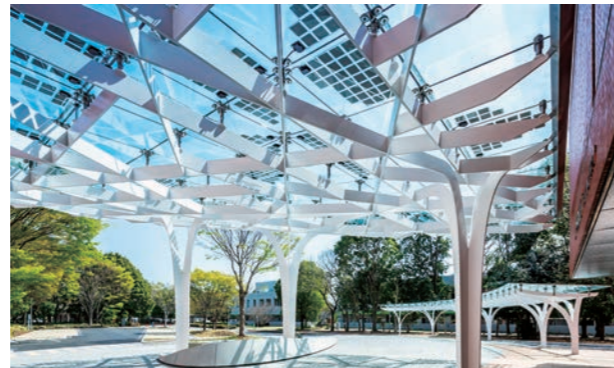
A tree-shaped entrance canopy was installed in front of the main building to portray solar panel installation, research progress, and growth as a symbol of a carbon-free society
