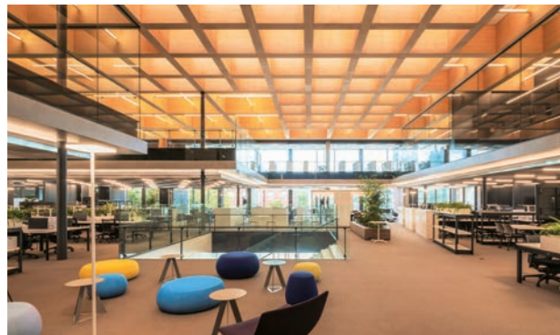
Roof frame structure which supplies soft natural light to workspaces
