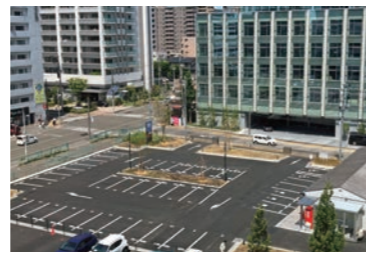
PET Ascon, which uses discarded plastic bottles (Parking lot of Tohoku Branch Office Building, Shimizu Corporation)
