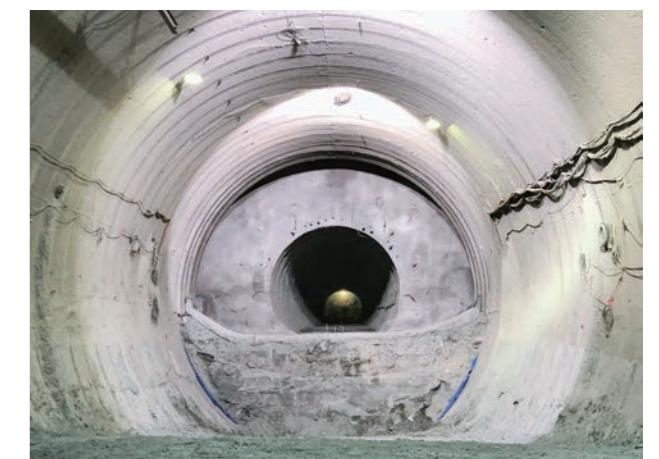
Cross-section closure of main tunnel in center drift advancing method Otonaka tunnel excavation work in Otoineppu Village on National Route 40 (Otoineppu Village to Nakagawa Town in Nakagawa District, Hokkaido)
