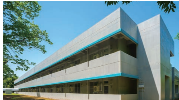
West-4A building, which achieved ZEB through renovation work
