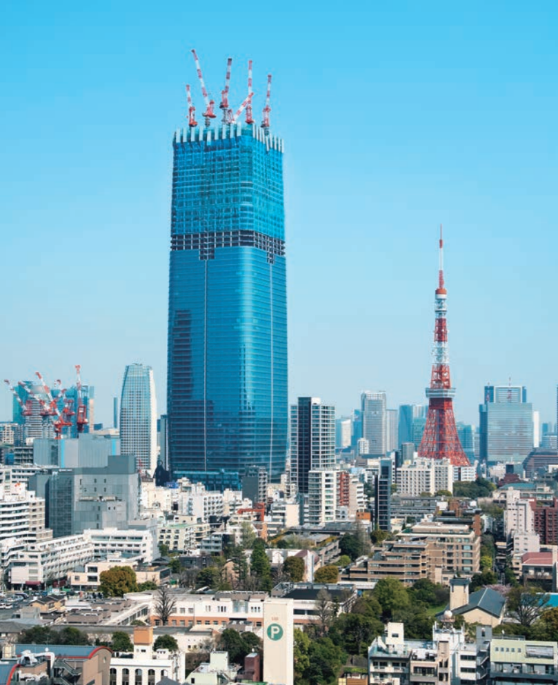
The A district of the Toranomon-Azabudai District Category 1 Urban Redevelopment Project (Minato ward, Tokyo)
