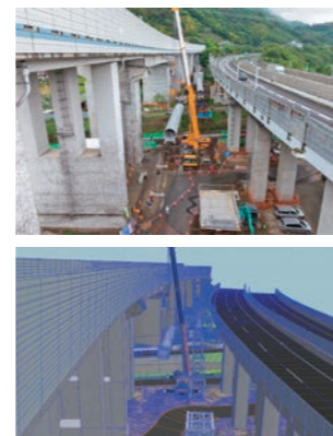
Actual construction site (top) and 3D construction simulation (bottom)
