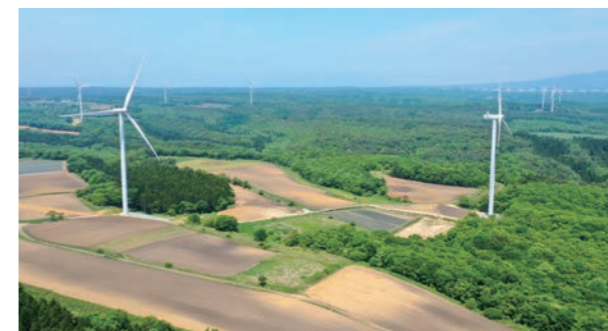
ReENE Rokkasho-Mura Wind Power Plant (Rokkasho-mura, Kamikita-gun, Aomori)
