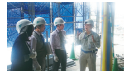
Construction site inspection (on-site inspection)
