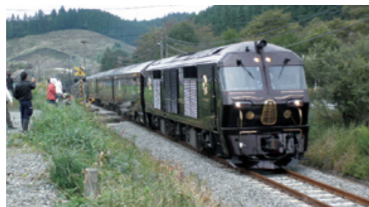
The Nanatsuboshi train passing through the restored Sakanoue Tunnel (at rear left)
