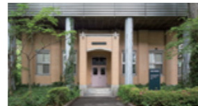
Musashi University Ekoda Campus From left: Building No. 3 (new design/construction, remodeling) Large lecture hall (new construction, remodeling) Nezu Chemical Laboratory (new construction, remodeling)
