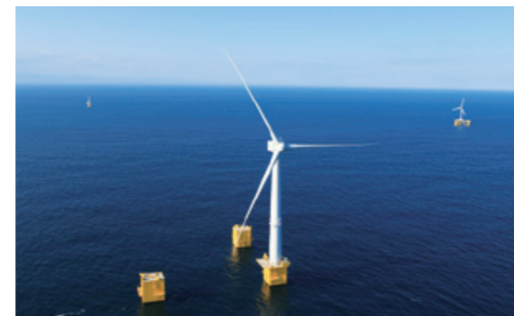
Fukushima Restoration and Floating Offshore Wind Farm Contracted by the Ministry of Economy, Trade and Industry to a consortium of 11 companies (including Shimizu)
