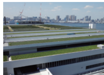
Rooftop landscaped garden
