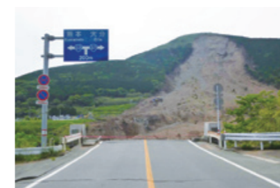
A landslide near Aso Ohashi Bridge
