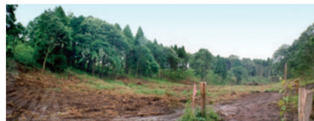
Utilizing existing valley to build foundations for waterscape
