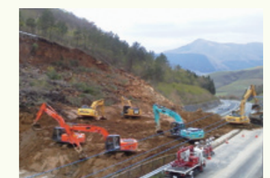
Emergency repairs to Oita Expressway
