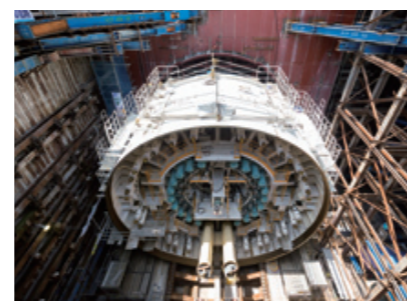
The entire shield machinery
