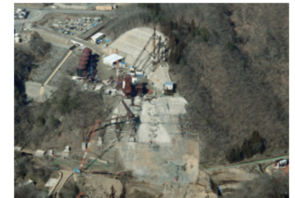
Construction of the Yanba Dam main structure (Gunma Prefecture)
