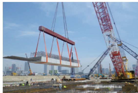
On-site PC construction helped reduce labor requirements.
