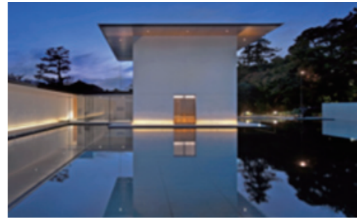
D.T. Suzuki Museum (construction) (Photo courtesy of D.T.Suzuki Museum)
