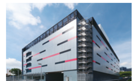
1-Net North Data Centre (Singapore)
