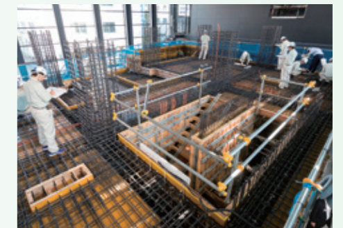
Training for reinforced concrete inspections
