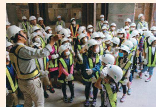
Students from a school for children of Japanese expatriates touring the construction site
