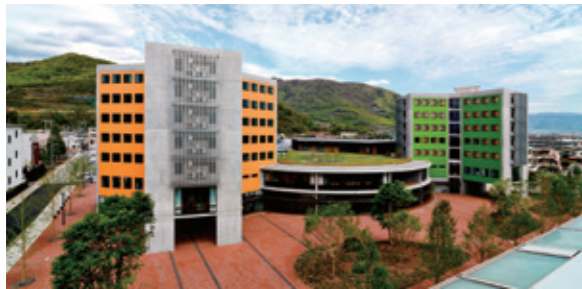
Yamanashi Gakuin University International College of Liberal Arts (design/construction [joint design])
