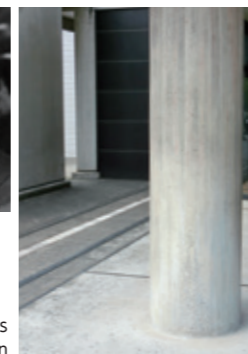
A pilotis pillar that retains its original wood grain
