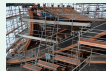
Dismantling work and research under way beneath the temporary roof
