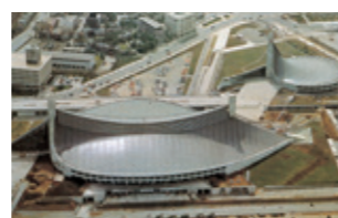
Yoyogi National Stadium
