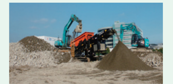
Reusing rubble from a large-scale demolition project
