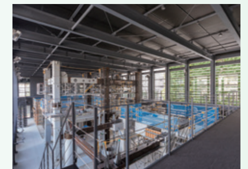
The precast (PCa) zone
