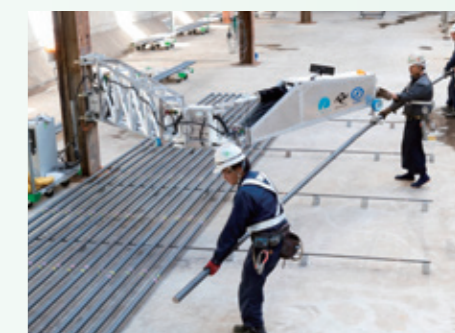
Testing the rebar arrangement assistant robot
