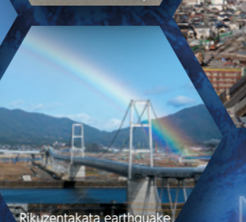
Rikuzentakata earthquake restoration project
