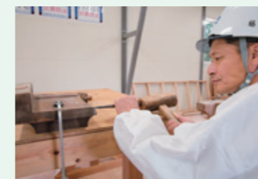
A temple carpenter working on shrine repairs
