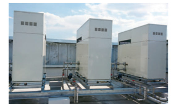
TMG Asaka Medical Center (Asaka, Saitama Prefecture) Achieved Energy Conservation and BCP in Energy Services for Cogeneration Systems
