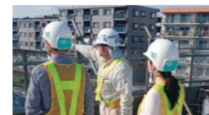
Construction site inspection (on-site inspection)
