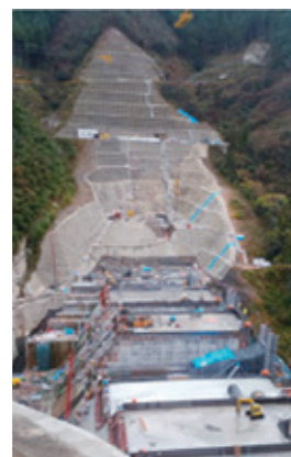
Hirase Dam (Iwakuni, Yamaguchi Prefecture)
